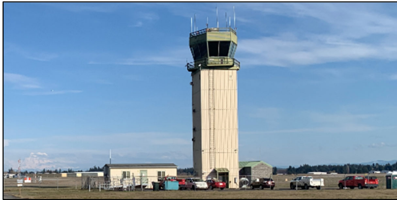
Figure 1-14: OLM Air Traffic Control Tower
