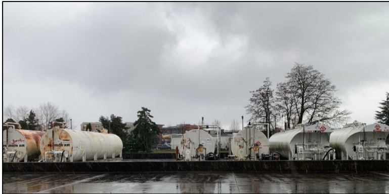
Figure 1-15: OLM Fuel Storage Area
